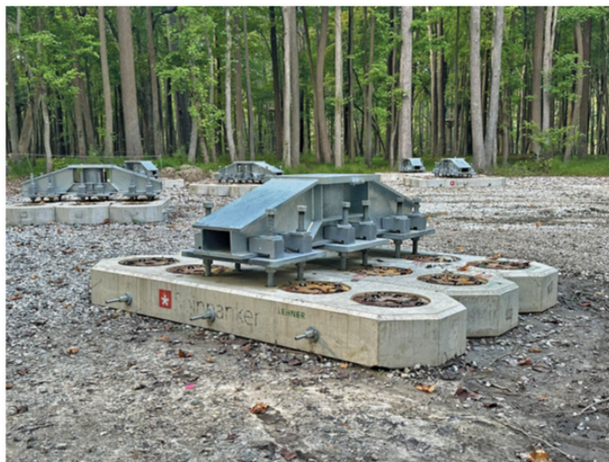
The precast foundation technology deployed is modular, so multiple elements can be tied together to create anchor points.
